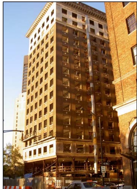
The Ellis under Construction in the Westside TAD
