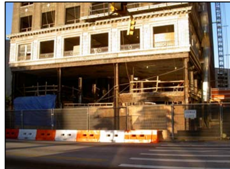
The Ellis under Construction in the Westside TAD
