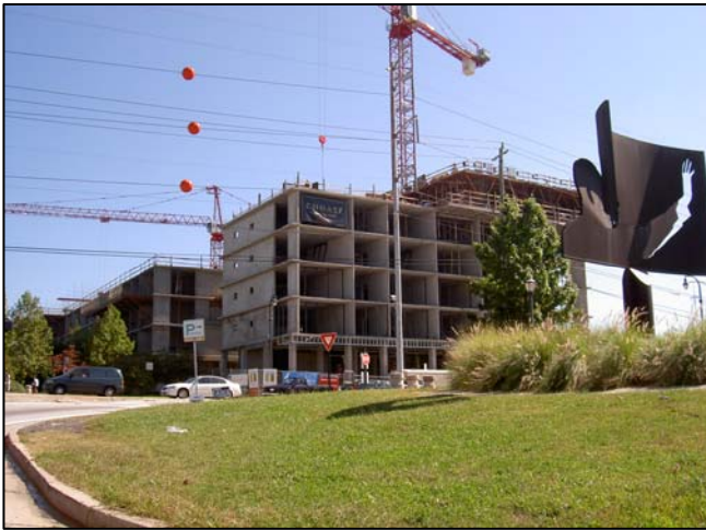
Tribute Lofts under Construction in the Eastside TAD
