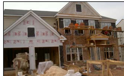
Single-Family Home Under Construction
