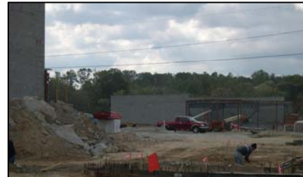
Retail Under Construction
