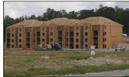
Apartments Under Construction
